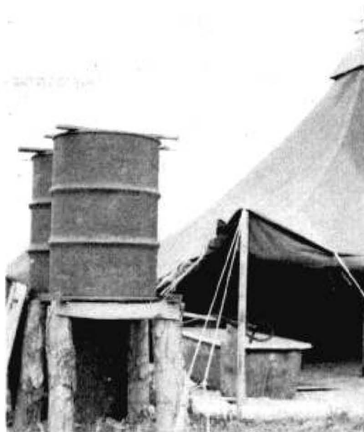
Improvised Bath House. The water is heated by the sun.
